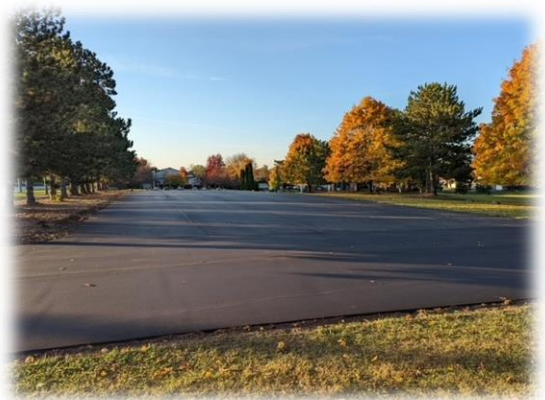
Smooth new pavement - Taft Road parking lot
